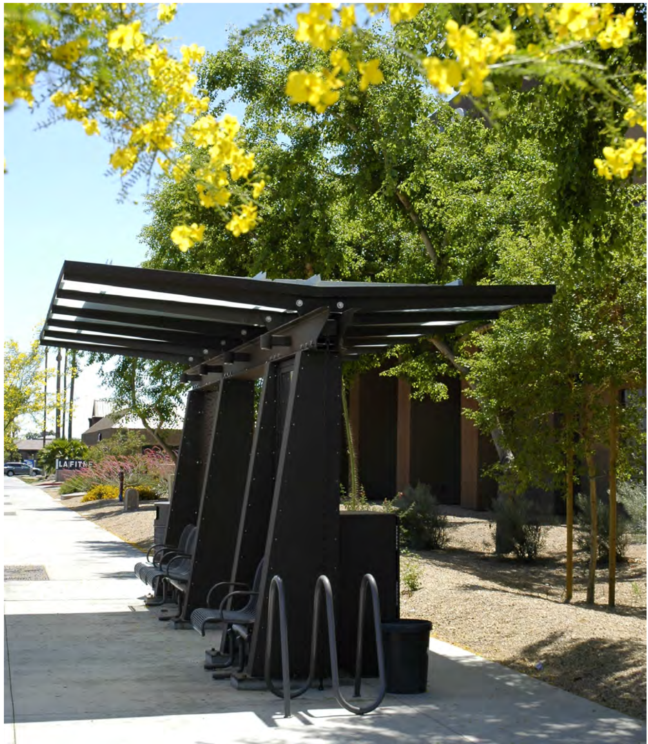
Transit shelter designed by Otak, Inc. for the Scottsdale Road Corridor in Scottsdale, Arizona using the Kit of Parts approach—note that the roof incorporates solar photovoltaic panels for to generate energy for lighting
