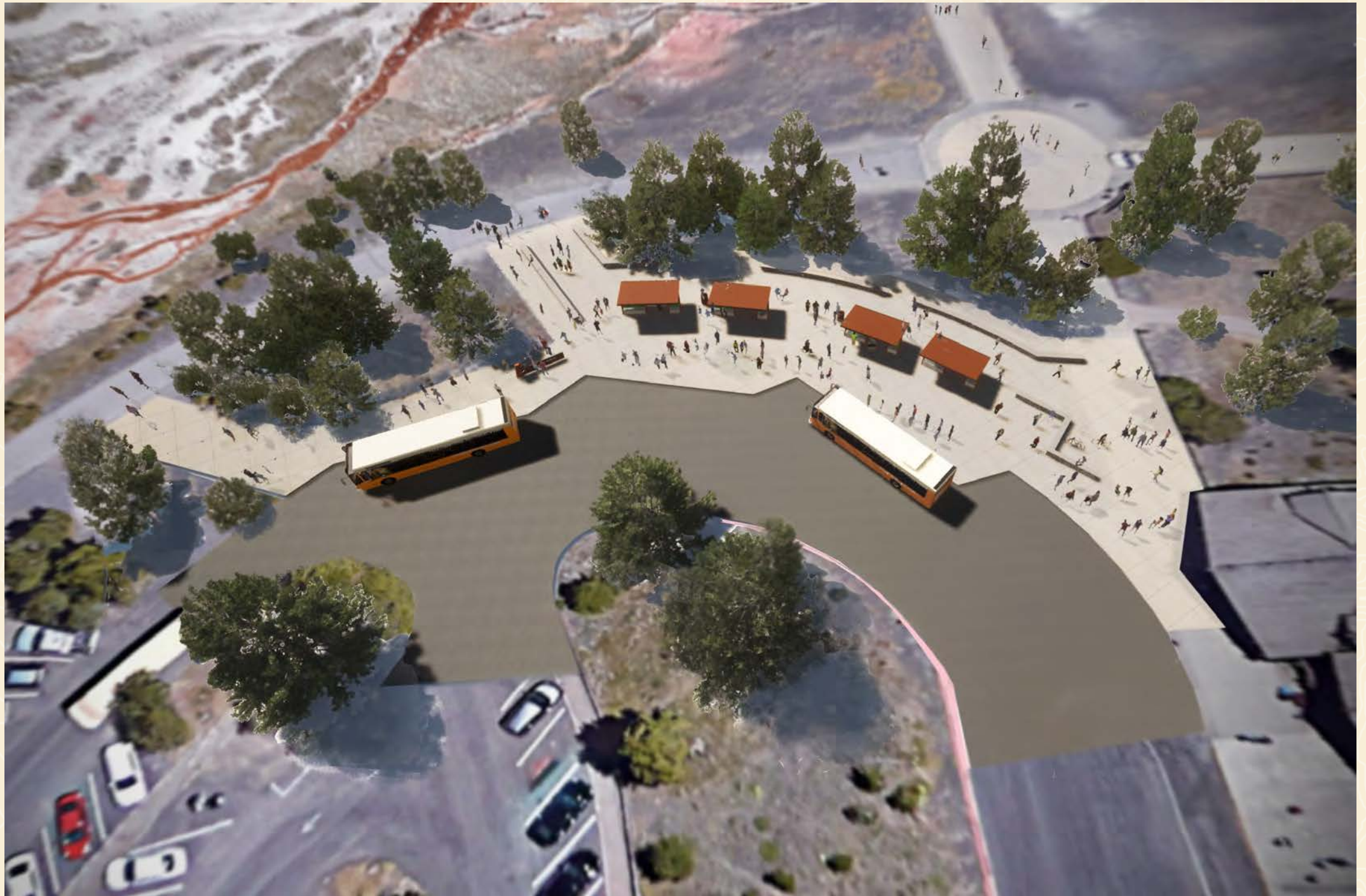
Figure 7.26—Bird's Eye Perspective Rendering of the Old Faithful Shuttle Terminal, Note Sawtooth Bus Bay Configuration
