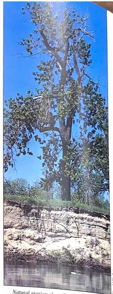
Natural erosion along the Bismarck segment.
