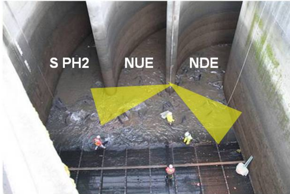
Figure 35. Photo of the dewatered Bonneville junction pool, showing JPN (left triangle) and JPW (right triangle) DIDSON deployments and the three routes that upstream migrants use to enter the pool (NDE, NUE, and S PH2).
