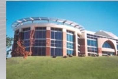
Bruker Corporation Headquarter Billerica, Massachusetts, USA
