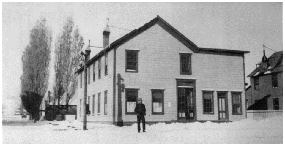
Cassia County Courthouse located in Albion Idaho (county seat until 1919)
