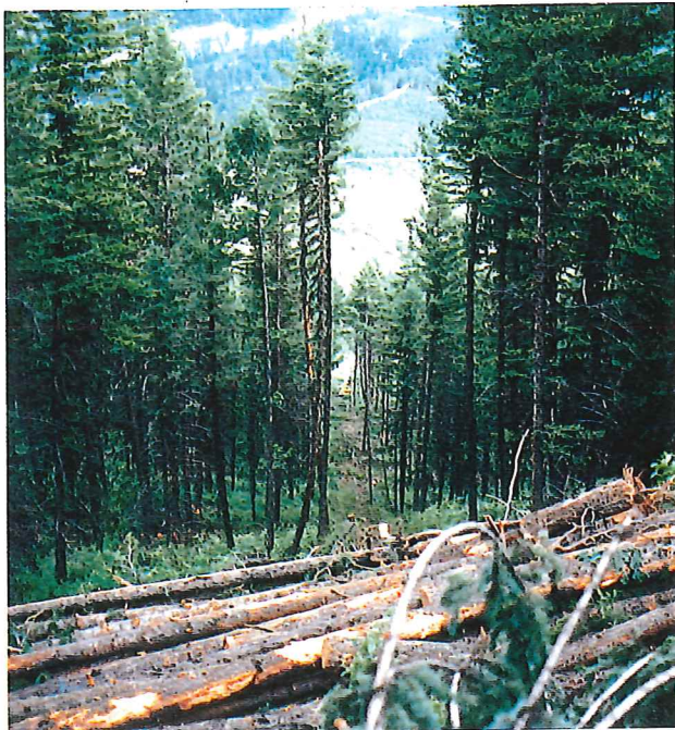
Skid trail with a Skyline system.
