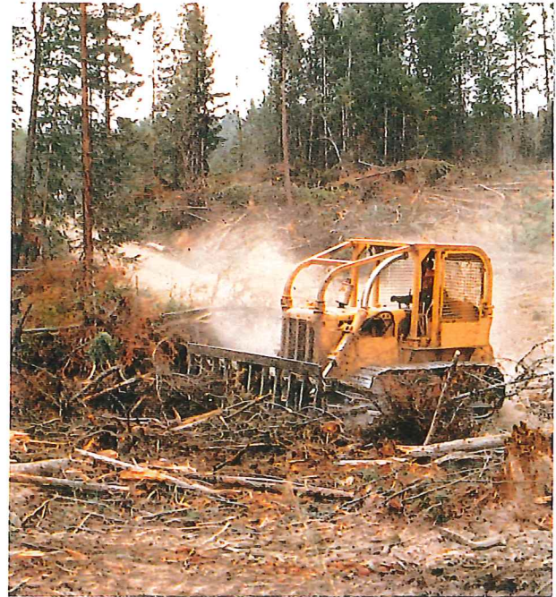
Mechanical scarification used here will prepare this site before planting.
