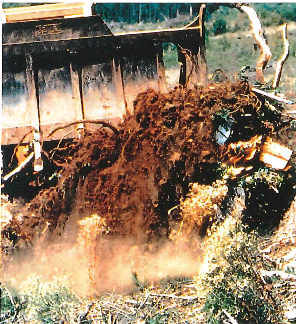
Piling and burning logging slash reduces fire hazard and the potential for beetle infestation. Above, too much soil is being moved with the slash.
