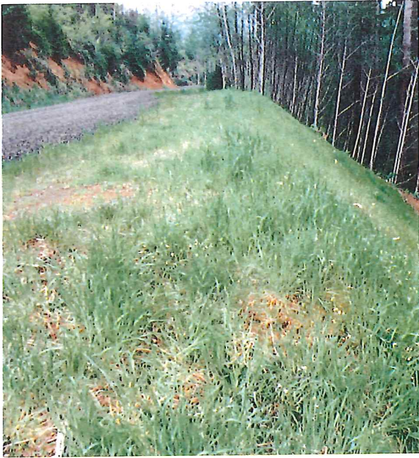
Seeding grass will help prevent erosion.
