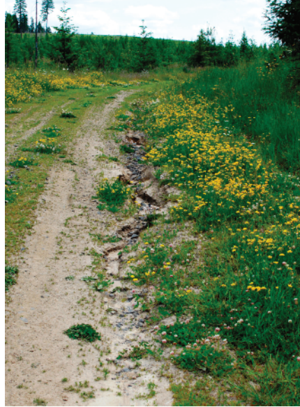
When the amount of water from precipitation and/or snowmelt exceeds soil infiltration rates, water flowing over exposed mineral soil surfaces can cause surface erosion.
