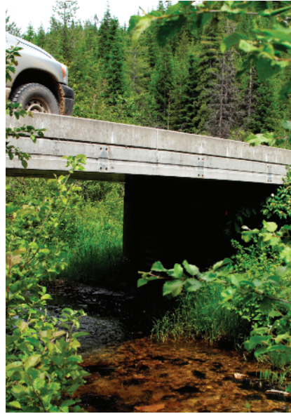
Bridges provide the best fish passage, have longevity, and require minimal maintenance.
