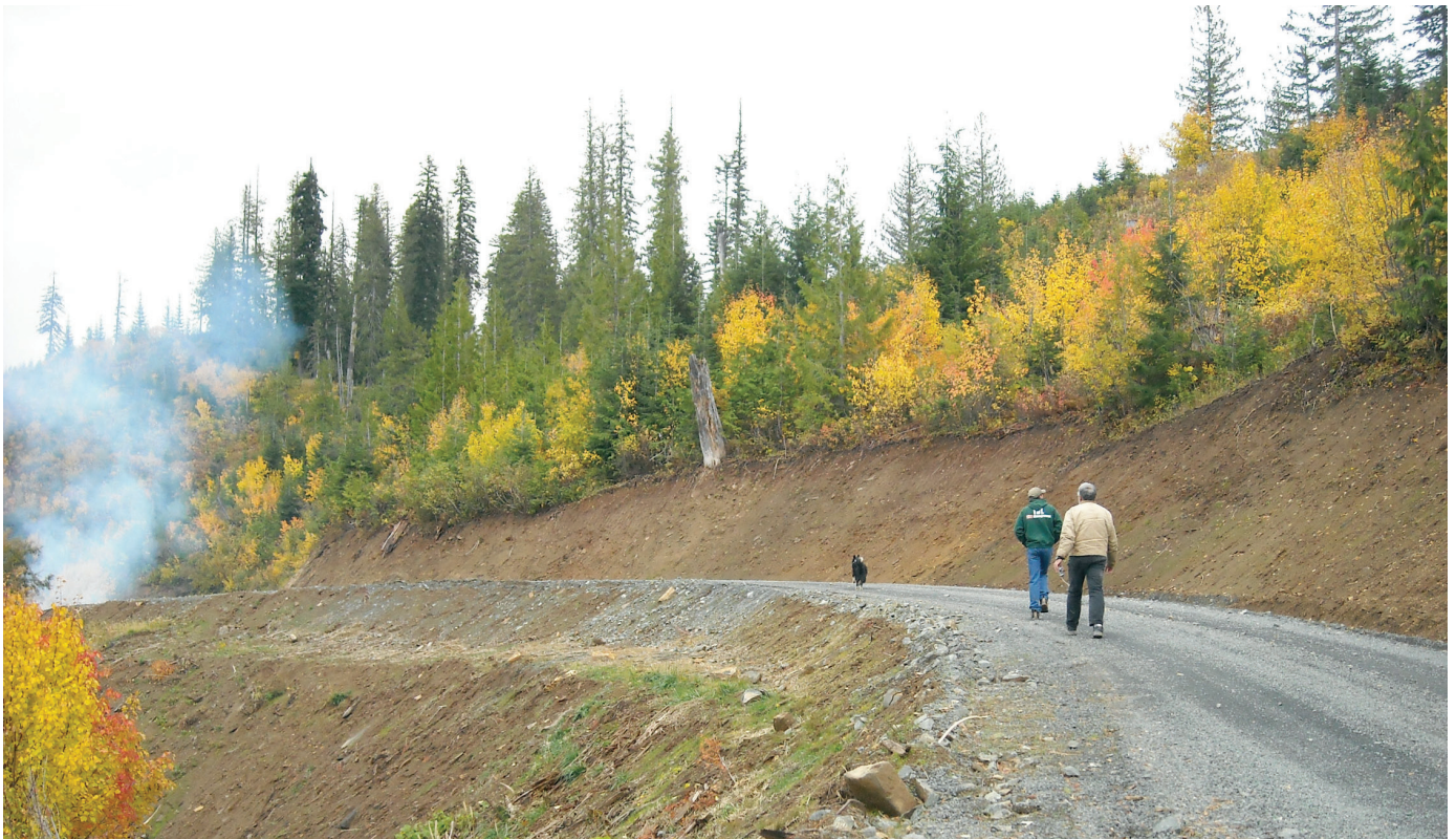
Forest roads built on steep slopes, erodible soils, or stream crossings hold the greatest potential for degrading water quality.
