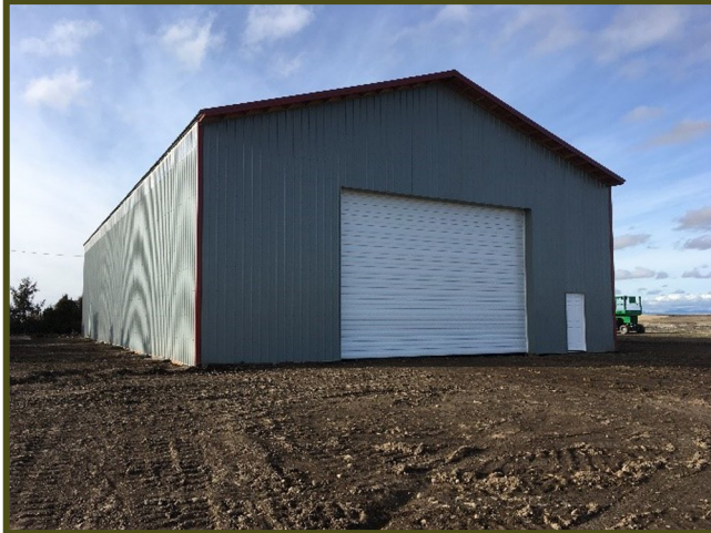
The new shed at WSU Wilke Research and Extension farm.
