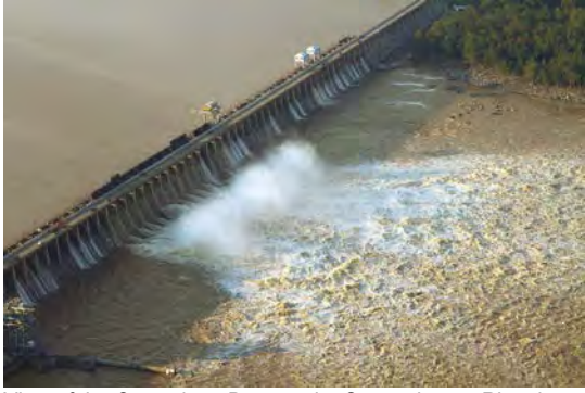
View of the Conowingo Dam on the Susquehanna River in the aftermath of Tropical Storm Lee. Photo taken at 4:30 p.m., September 12, 2011. Discharge at time of the photo was 220,000 cubic feet per second. Peak discharge for the flood was 778,000 cubic feet per second at 4:00 a.m. on September 9, 2011. (Photo by Wendy McPherson, USGS; Figure from Hirsch 2012)
