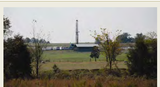
“On-the-ground” USGS projects, designed with Cooperators and partners, are proposed or ongoing in more than 15 States that monitor and assess possible impacts of energy production on water resources. Photo shows hydraulic fracturing operation in the Fayetteville Shale Formation on a farm in Arkansas. (Photo by Bill Cunningham, USGS)
